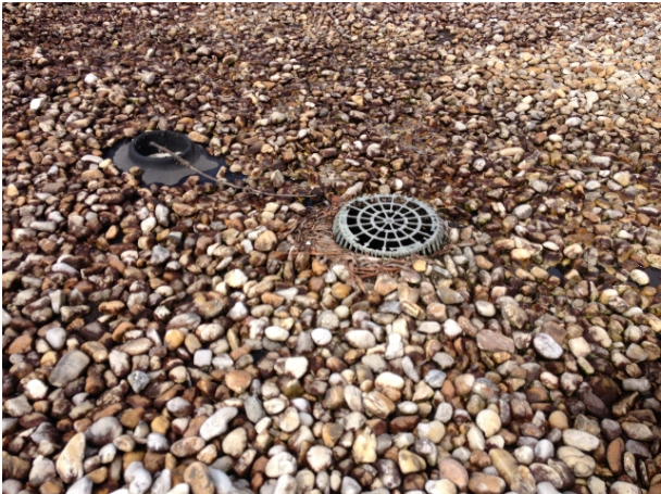
Drain and over flow drain
