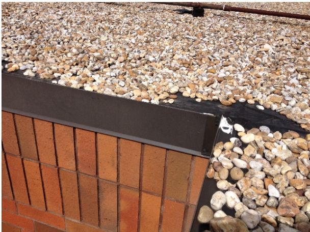
Gravel stop detail at perimeter
