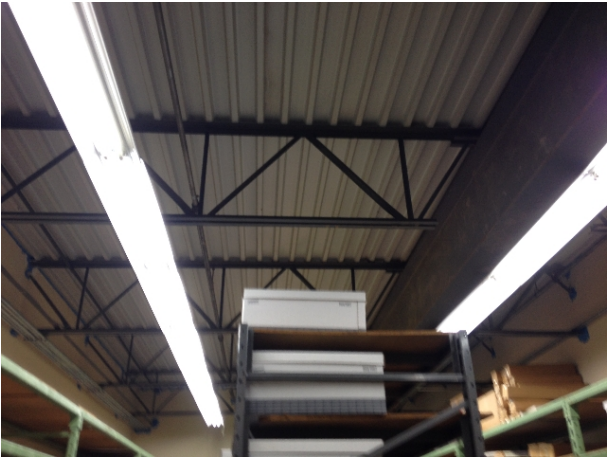
Photo of underneath side of decking
