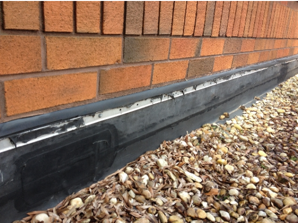
Termination bar detail at high walls
