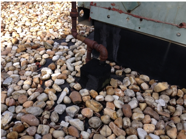
Typical pitch pan at HVAC unit
