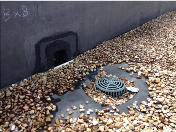
Drain and scupper detail
