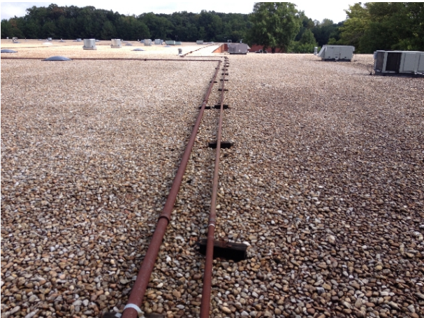
Rusted pipes on roof (recommend painting in future)
