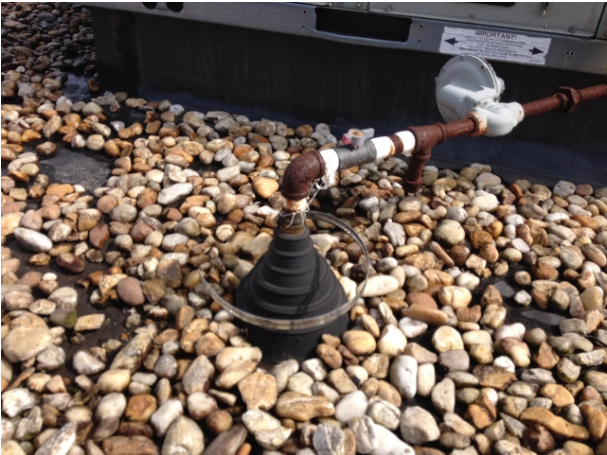
Typical pipe boot flashing at unit
