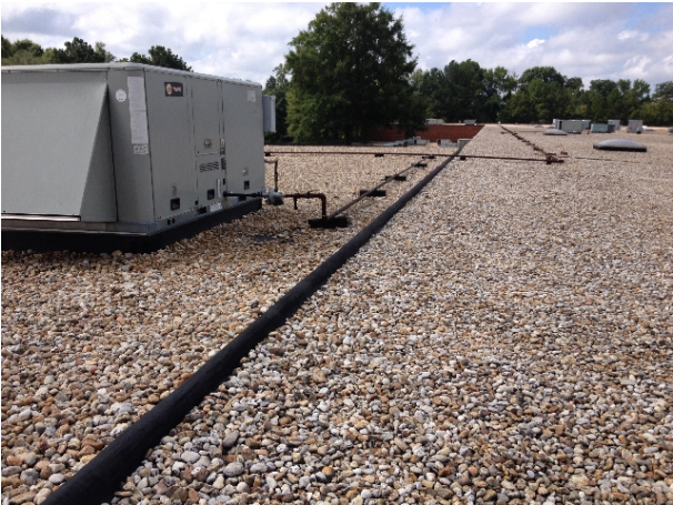
Expansion joint at front area
