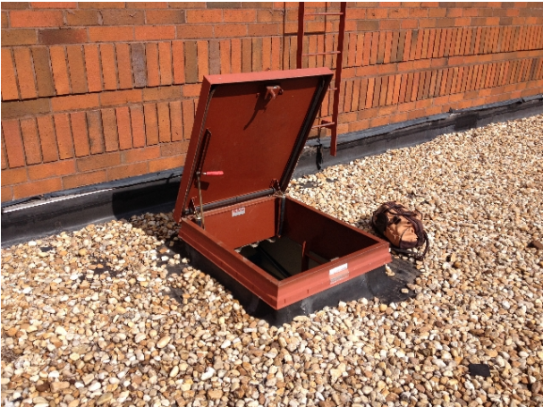
Roof hatch access to roof
