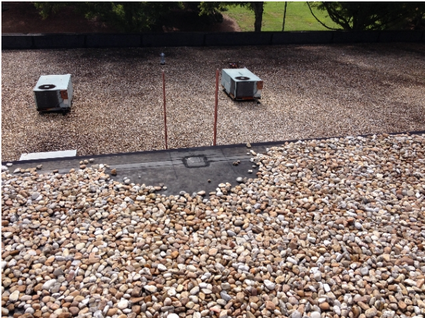
Ladder access to roof (needs walk pad)
