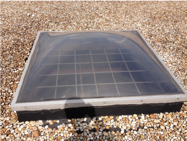
Safety/burglar bars mounted on inside of skylight
