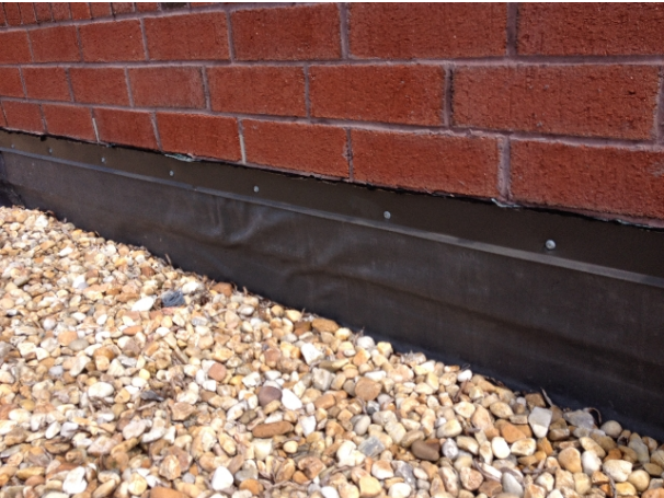
Typical Flashing Detail
