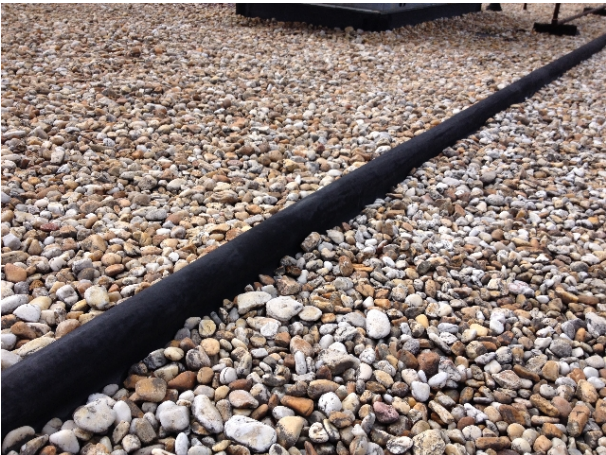
Close up of expansion joint
