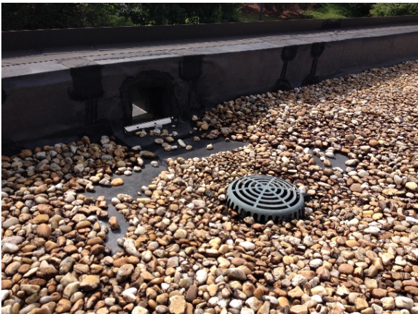
Photo of front wall wrapped with drain and scupper
