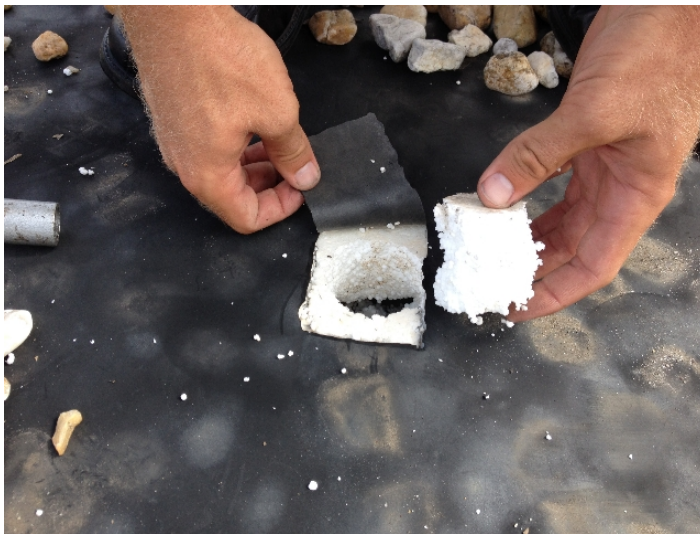
Test Cut 2 EPDM-Ballast 2" EPS Metal Deck
