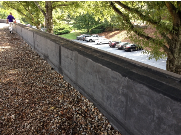
Outer parapet wall wrapped in membrane
