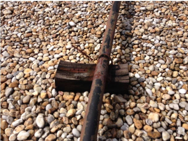
Wood blocking at pipes in bad condition (many are not fastened anymore)
