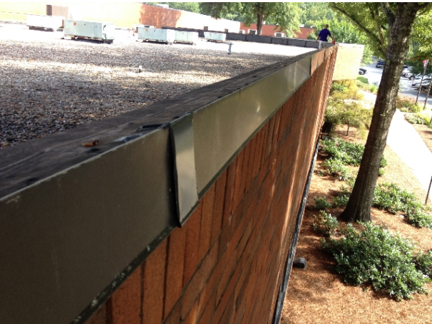
Gravel stop edge metal on parapet
