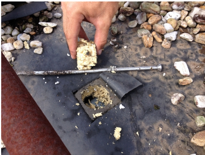
Test Cut 2 (New Extension) EPDM-Ballast 1.5" PolyIso Metal Deck
