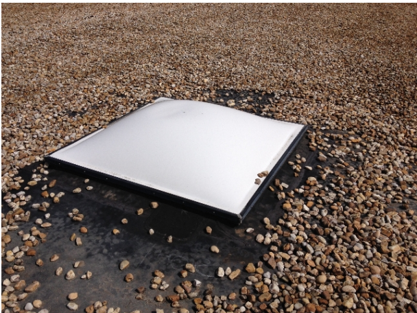
Skylight that is completely white
