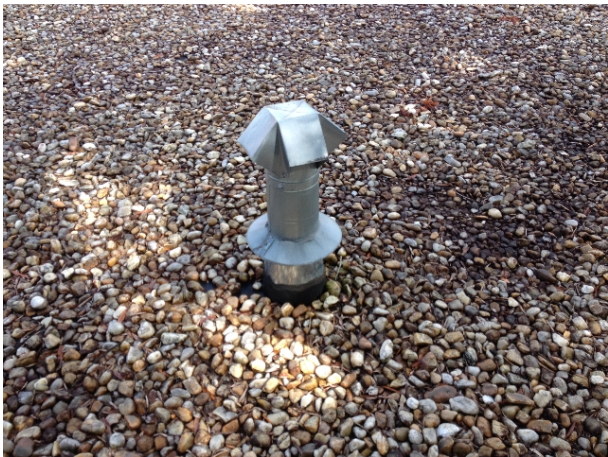
Typical roof vent
