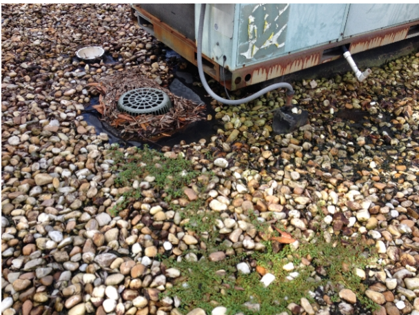
Drain and over flow drain pipe acting as drainage for roof (3 sets)
