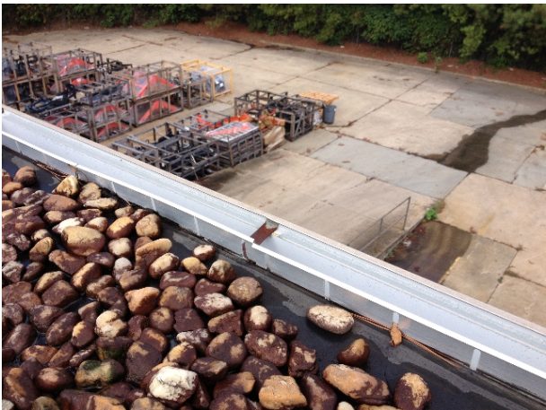
Gravel bar at gutter
